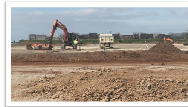
Ground works FEB 2016
